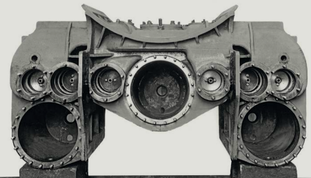
The original monobloc cast iron cylinder block for No. 2001 Cock o’ the North (front view).
